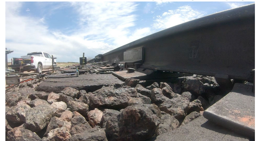
Location C: Poor Support (40 mph)
