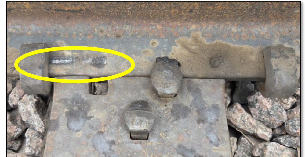
Rail slide through anchors
