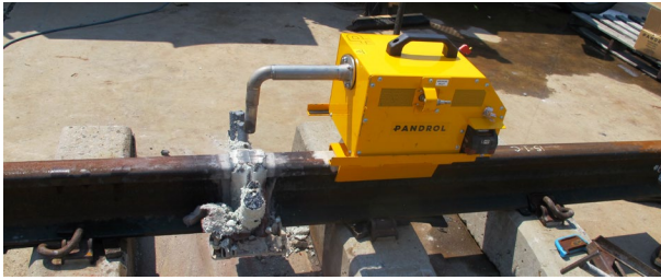
Figure 7. HFP using air quenching to cool a thermite weld
