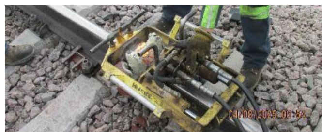
Figure 6. MxV Rail shear used during head repair trials
