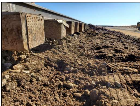
Test Section after Shoulder Cleaning
