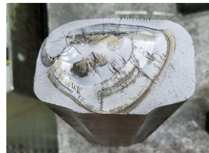
Transverse defect in rail
