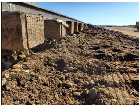
Test Section after Shoulder Cleaning
