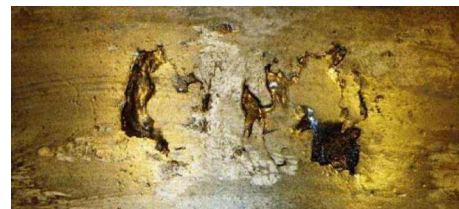
Wheel tread spalling
