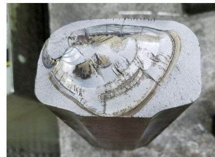
Transverse defect in rail
