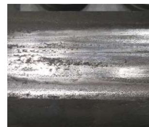
Pitting on wheel tread (top) and rail surface (bottom) due to water
