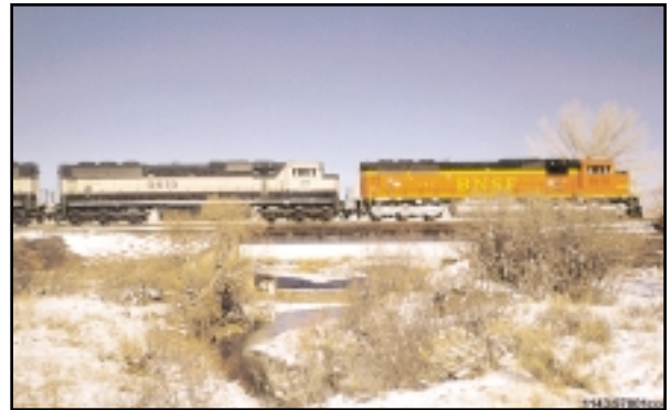
Exhibit 1. BNSF Bridge at Barela, Colorado
