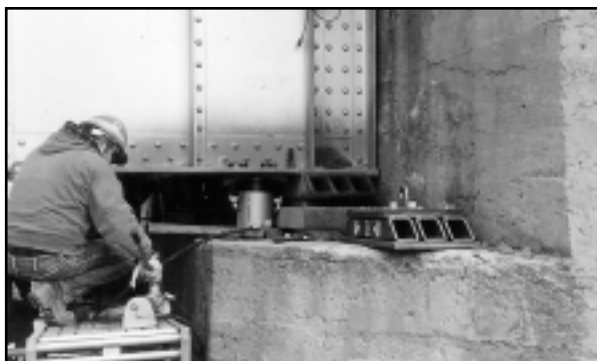
Exhibit 2. Installing Instrumented Bridge Bearings
