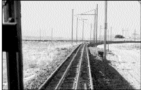
Exhibit 2. Curved Section of Track on the Rail Defect Test Facility
