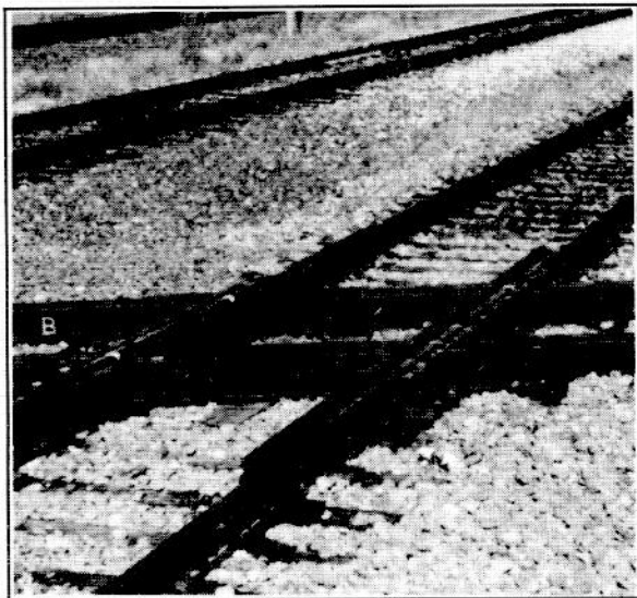
Exhibit 1. 62-degree Three-Rail Crossing
