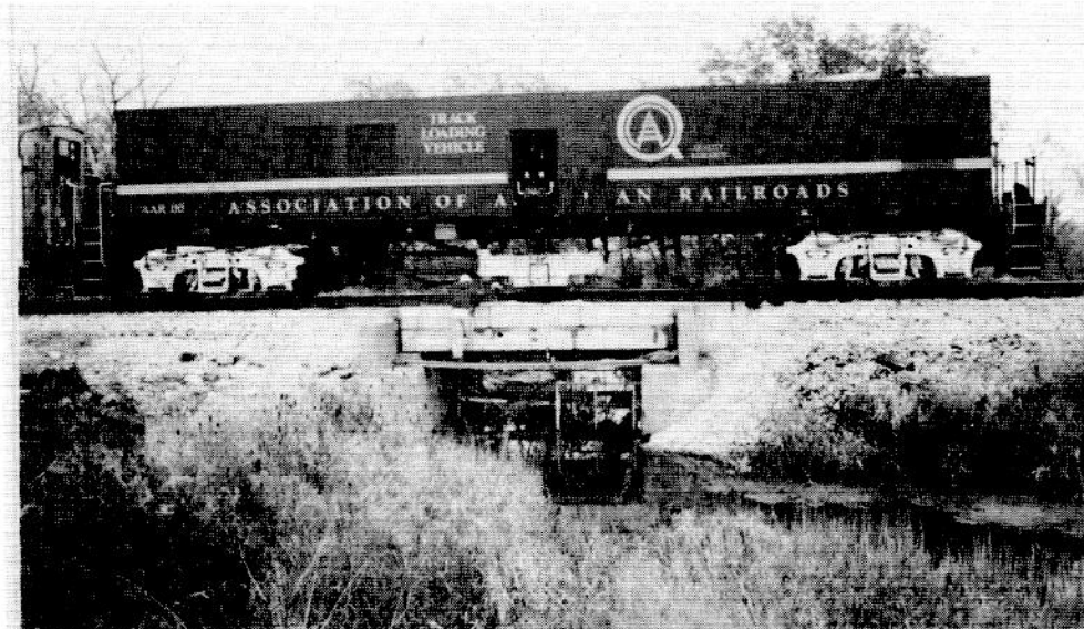
Exhibit 1. AAR's TLV Loading the Concrete Bridge.
