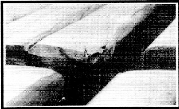
Exhibit 3. Crossing Rail End after 4.6 MGT of HAL Traffic
