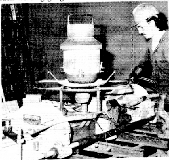
Exhibit 5. Typical Rail Puller Arrangement.
