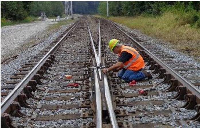
Figure 2. Kings Mountain, KY test location
