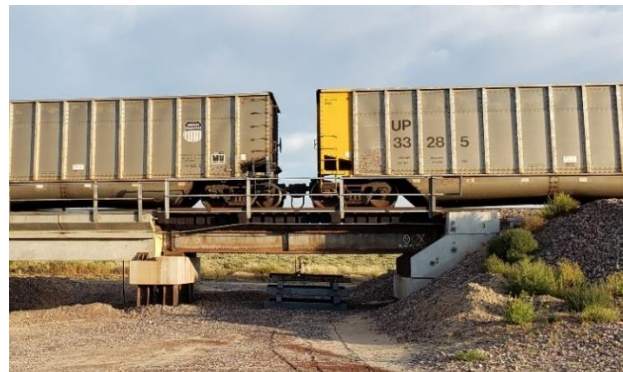
Figure 1. 30-foot riveted deck plate girder span at FAST
