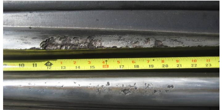
Figure 2. Wing running surface damage at South Fork test frog location
