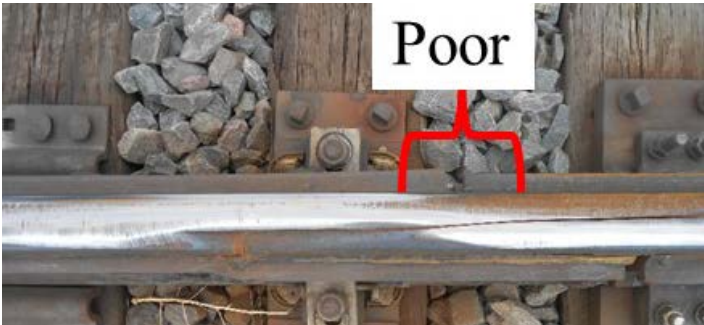
Figure 4. Poor wheel transfer zones on LAP IJs
