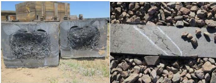
Figure 1. Center cracking of EPC ties
