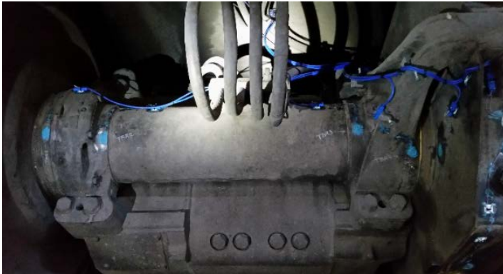
Figure 3. Thermocouples were placed on select components.
