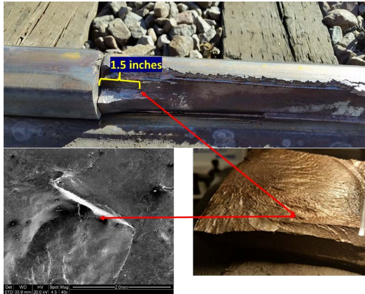
Figure 4. Fatigue defect at various magnifications
