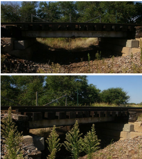
Figure 2. Bridge 209.22 I-Beam span near Kirkland, Texas
