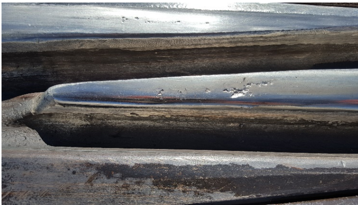
Figure 2: Chipping of laser cladding frog after 23 MGT
