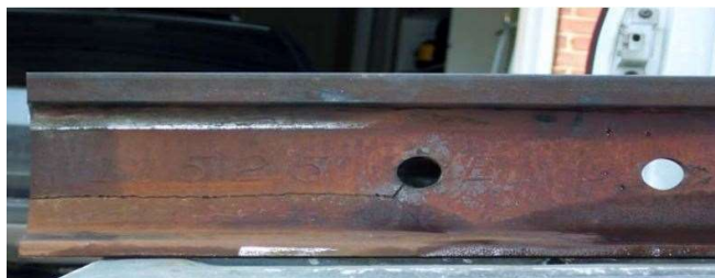
Figure 1. Bolt hole crack (BHC) defect 2
