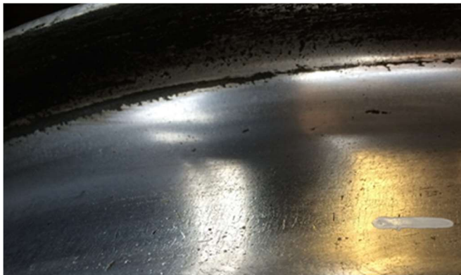
Figure 2. Fine surface cracks in an HPW after 430,000 miles. Wheelset currently has 480,000 miles.
