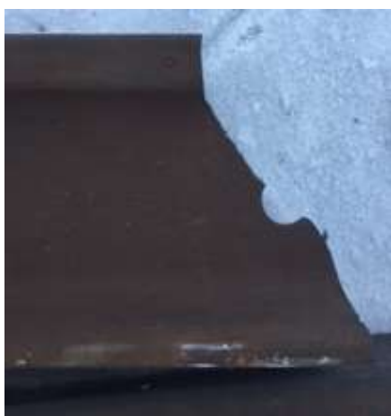
Figure 6. Example of fracture from a bolt hole
