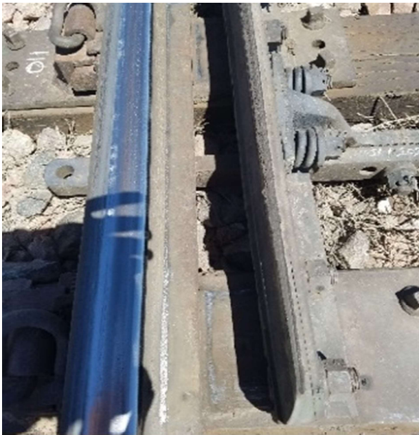
Figure 7. Switch Points with Brushes
