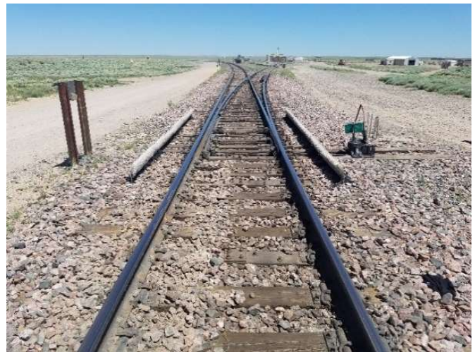
Figure 2. No. 10 Right-hand Turnout at FAST Looking East
