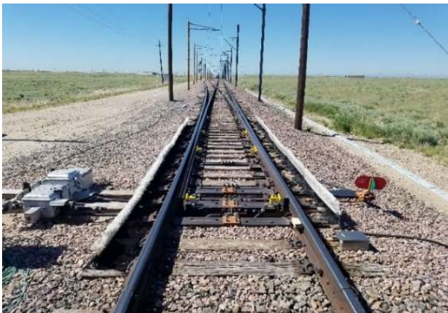
Figure 3. No. 20 Left-hand Turnout on RTT Looking South
