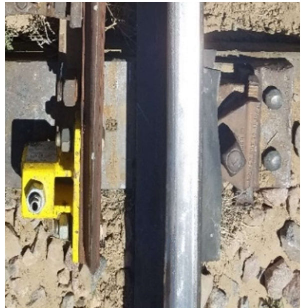
Figure 8. Switch Points without Brushes
