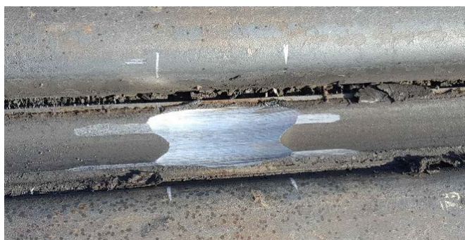
Figure 2 Simulated "New" OWLS Flangeway Gap Ground into Existing Coupon
