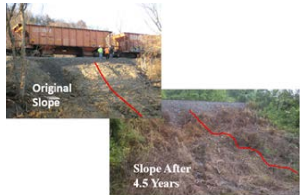
Figure 3: Comparison of planar embankment profile at installation and hummocky profile after 5 years
