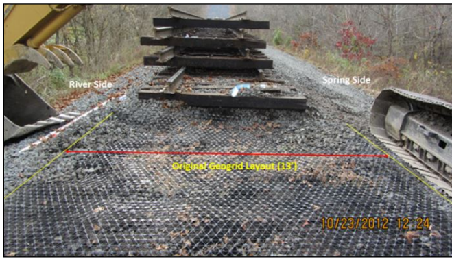
Figure 4: TX190L geogrid was symmetrically located under the ties during installation
