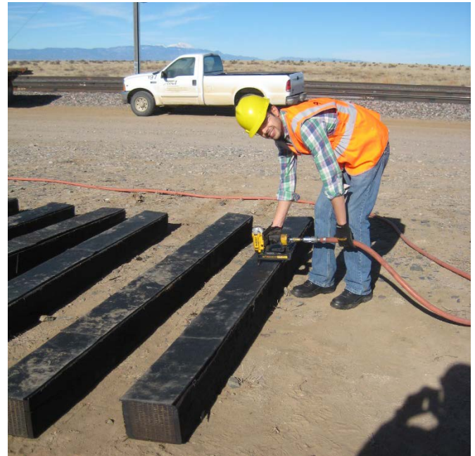
Figure 6. Under-tie Pads Being Attached to the Test Panel Timbers
