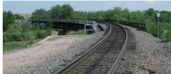
Figure 1. View of BNSF Bridge 617
