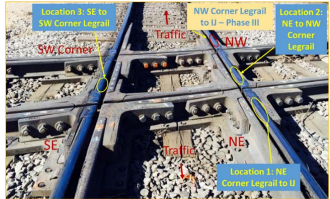
Figure 1. Rail break at the NW corner (red oval) at 59 MGT. The crossing diamond had been in service 100 MGT when a series of rail cracks were detected in the leg rails (yellow ovals)
