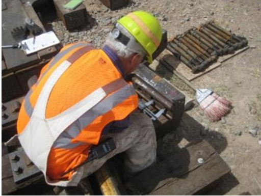
Figure 7. Measurement of bolt hole spacing
