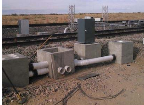
Figure 1. Installation of 3D TFDS foundations and conduits
