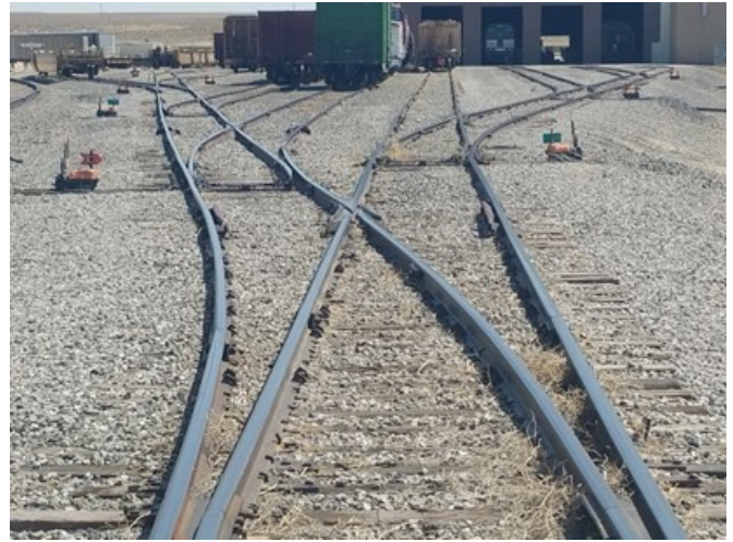
Figure 5. Typical Yard Ladder Track Arrangement
