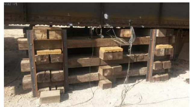
Figure 5. Safety Cribbing installed under 32-foot Span of FAST West Steel Bridge
