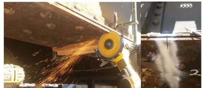
Figure 4. Three Notches Cut into Bottom Cover Plate of 32-foot Span South Girder
