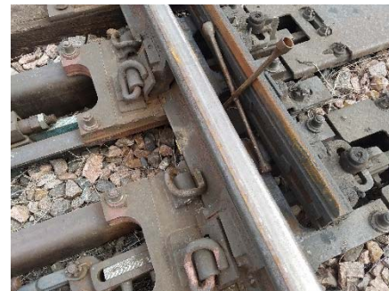
Figure 4. Foreign Object in Switch Point
