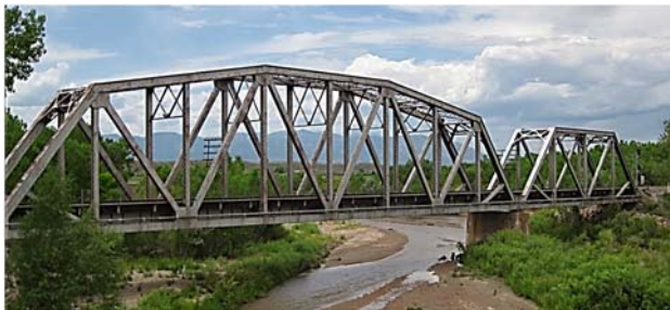
Figure 1. View of Bridge 93.94
