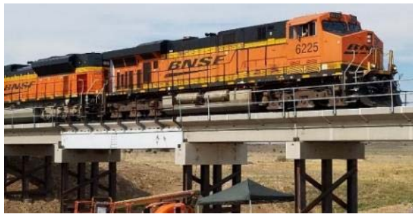
Figure 2. HCB Span on the BNSF Boise City Subdivision
