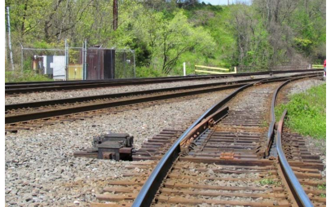
Figure 4. Typical Split Switch Derail
