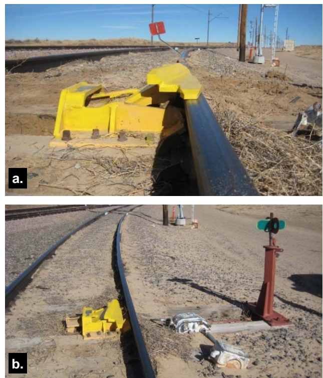
Figure 2. Typical Sliding Derail with Integral Crowder: a) Deployed, and b) Retracted
