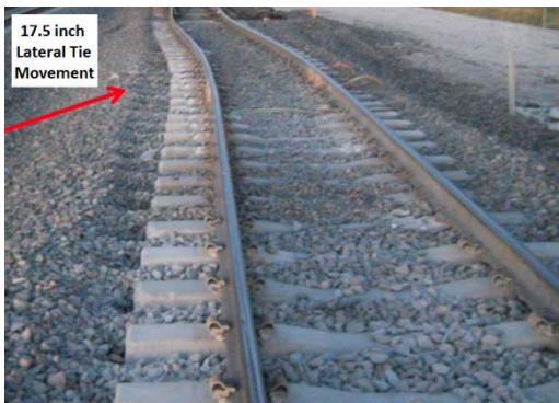
Figure 1. Track Panel Shift after Multiple Trains
