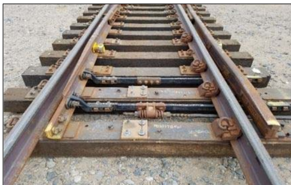
Figure 2. Vertical Lift Derail Panel
