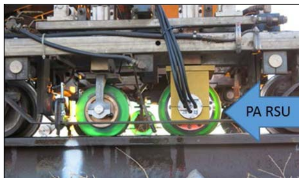
Figure 4. Phased Array RSU in Inspection Position
