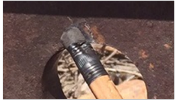
Figure 7. Bolt Hole Crack Defect on the RDTF
