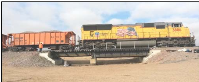
Figure 1. West Steel Bridge at FAST: 24-foot and 32-foot Riveted Deck Plate Girder Spans
