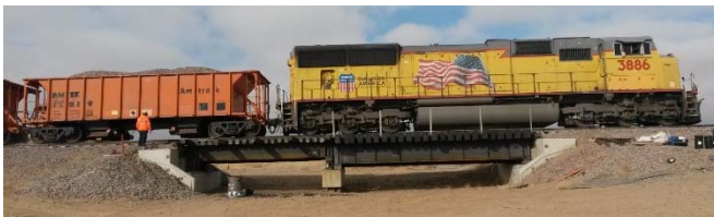
Figure 1. West Steel Bridge at FAST: 24- and 32-foot Riveted Deck Plate Girder Spans
