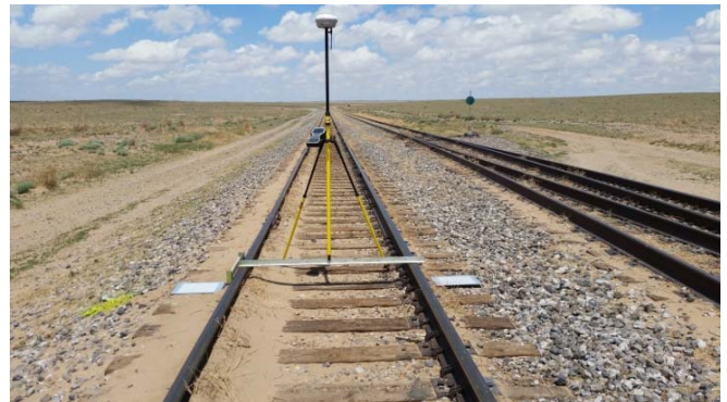
Figure 4. ALD to Define Test Zone and High Accuracy GPS Reading
