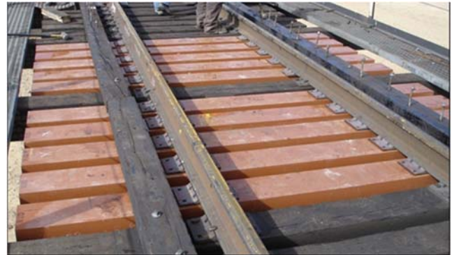
Figure 1. Bridge Tie Test on 55.5-foot Girder Span at FAST
