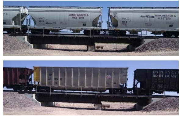
Figure 2. Short Cars (top) and Standard Length Cars (bottom) on Steel Bridge at FAST
