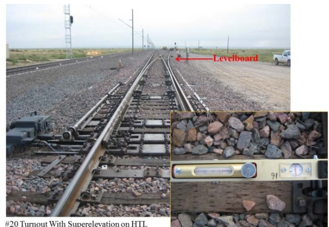
Figure 1. No. 20 Turnout with 0.5-inch Superelevation on the Diverging Route
