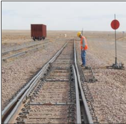
Figure 3. Presteered Switch (showing both mainline switch point and diverging stock rail)
