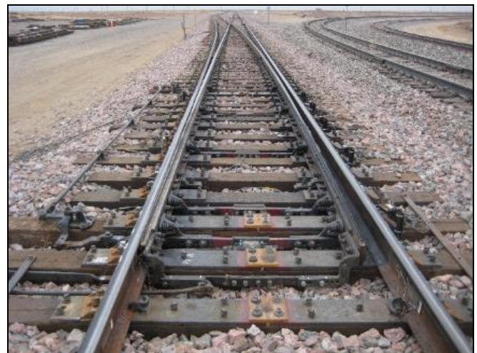
Figure 2. Prototype Presteered Switch No. 20 Turnout Installed at FAST
