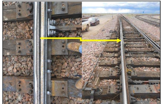
Figure 7. Diverging Stock Rail Wear and Running Surface Fatigue on Prototype Steered Switch
