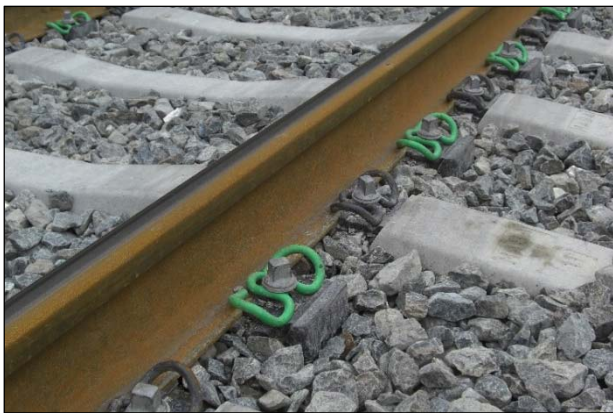
Figure 1. Crib Tie Test Zone on the ÖBB in Austria 1
