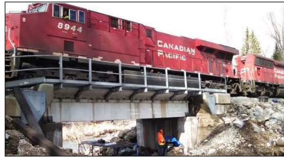
Figure 2: Bridge instrumented by TTCI for periodic measurements to observe long-term performance
