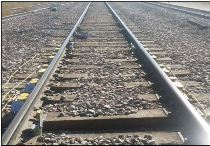
Figure 1. Broken rim detector system installed at TTC
