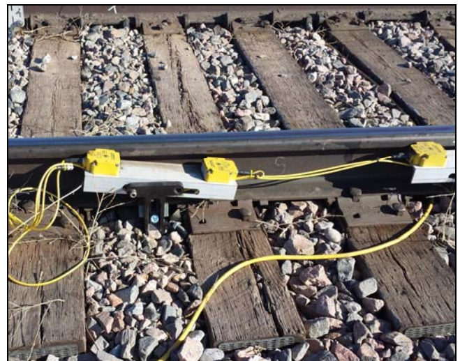
Figure 8. Unstable sensor brackets during testing at FAST
