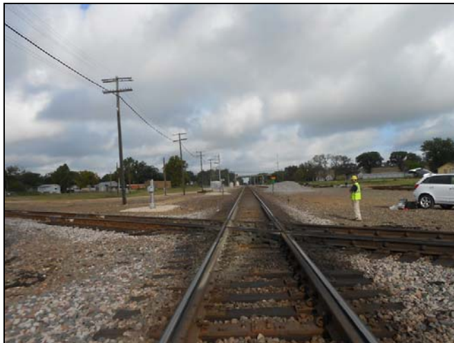
Figure 1. Full FBF Crossing Diamond Milano, TX
