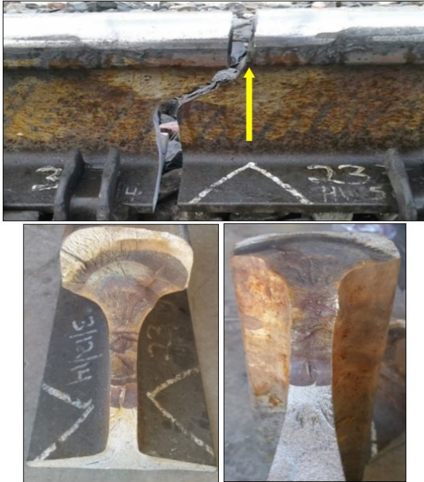
Figure 4. Weld Break, August 2014 (The yellow arrow points to the center of the HDR insert)
